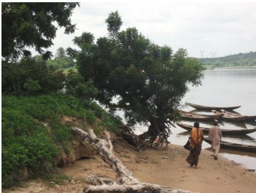
Photo 10.1: River Bank Erosion at Gungu Village
