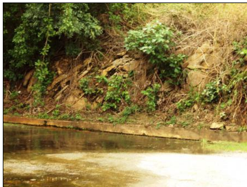
Photo 9.6: Side Wall Excavation to the Level Area Downstream of Drain AD53 (showing heavily jointed material).
