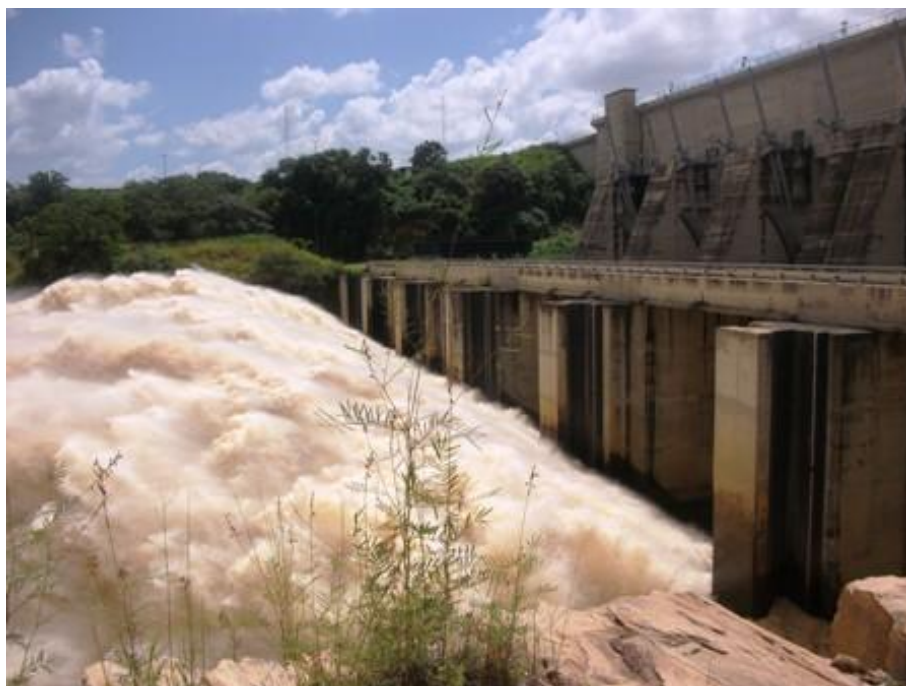
Photo 9.1: Flood Discharge Through the Spillway of Jebba Dam on 7 th Oct 2010
