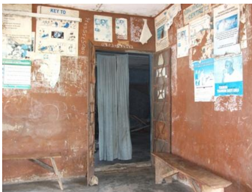
Photo 10.3: Primary Health Care Centre at Gungu Village
