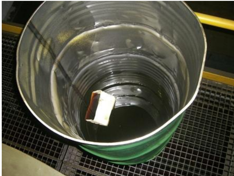
Photo 11.2: Unprotected Open Oil Drum
