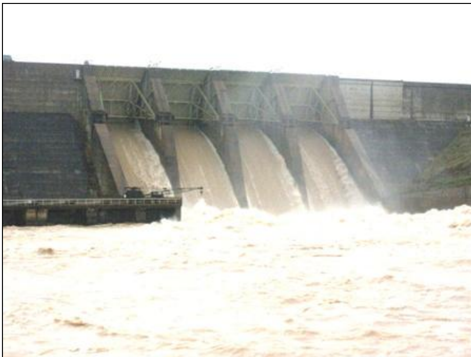
Photo 4.1: Discharge from Kainji Dam Spillway on 6 th October 2010
