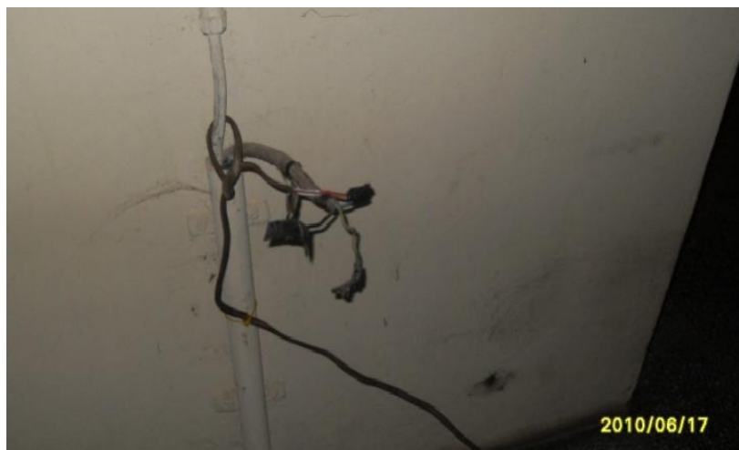
Photo 12.3: Exposed Wiring
