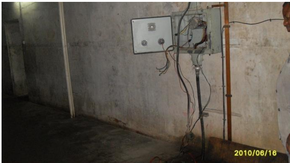
Photo 7.4: Exposed Wiring
