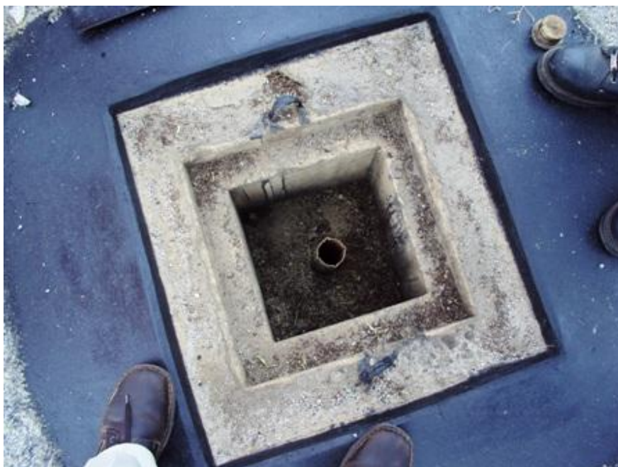
Photo 9.4: Headworks of Inclinator
